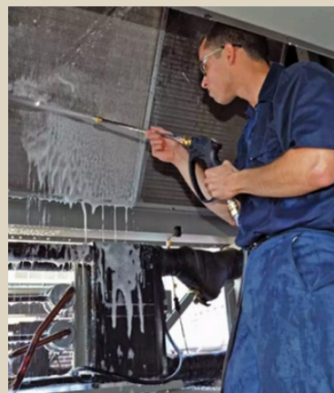
HVAC Condenser Cleaning
